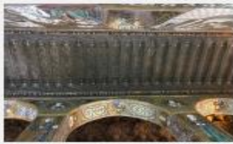
The ceiling with it's Muqarnas – an Arabic architectural detail that makes this chapel so unique with a blend of several styles
