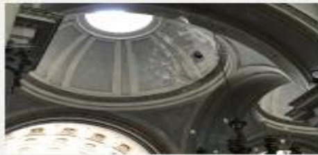
A Hole in the Dome to Let the Sun come Through to Align to the Meridian on the Cathedral's floor
