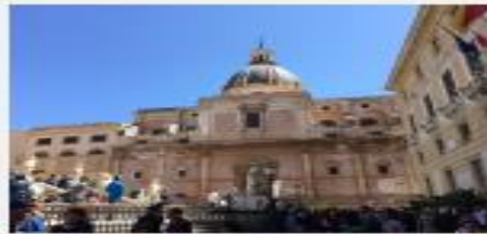
The Pretoria Fountain – Looking East; Santa Caterina is the church in back; on the left is the Cosma di Palermo
